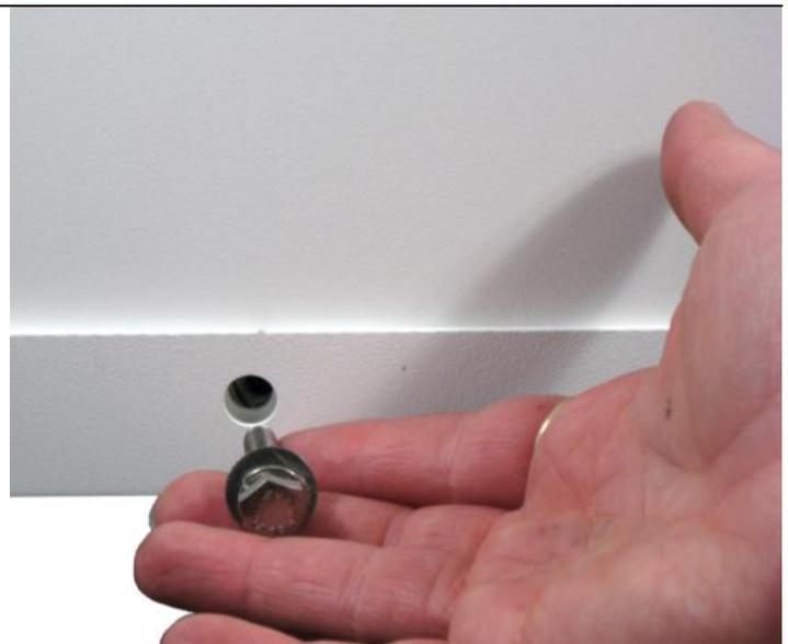
1. Remove the Aqua-Hot's access cover by locating the bolts securing it in place.
